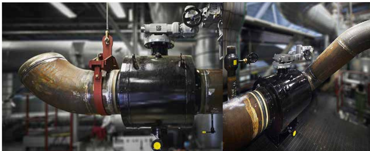
BROEN Ballomax® DN50 – Double bearing valve ball with Double Block and Bleed – DBB – outlet under the valve body
