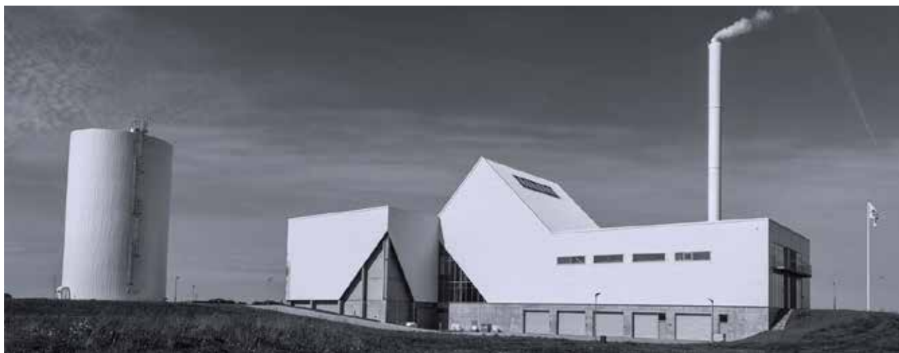
Aabybro district heating plant (Denmark).
