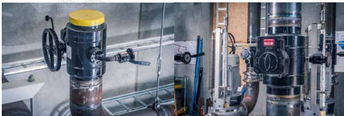
BROEN Ballomax® DN250 – DN400 valves – Double bearing valve balls with Double Block and Bleed and outlet – during welding at Hobro District Heating Station.
